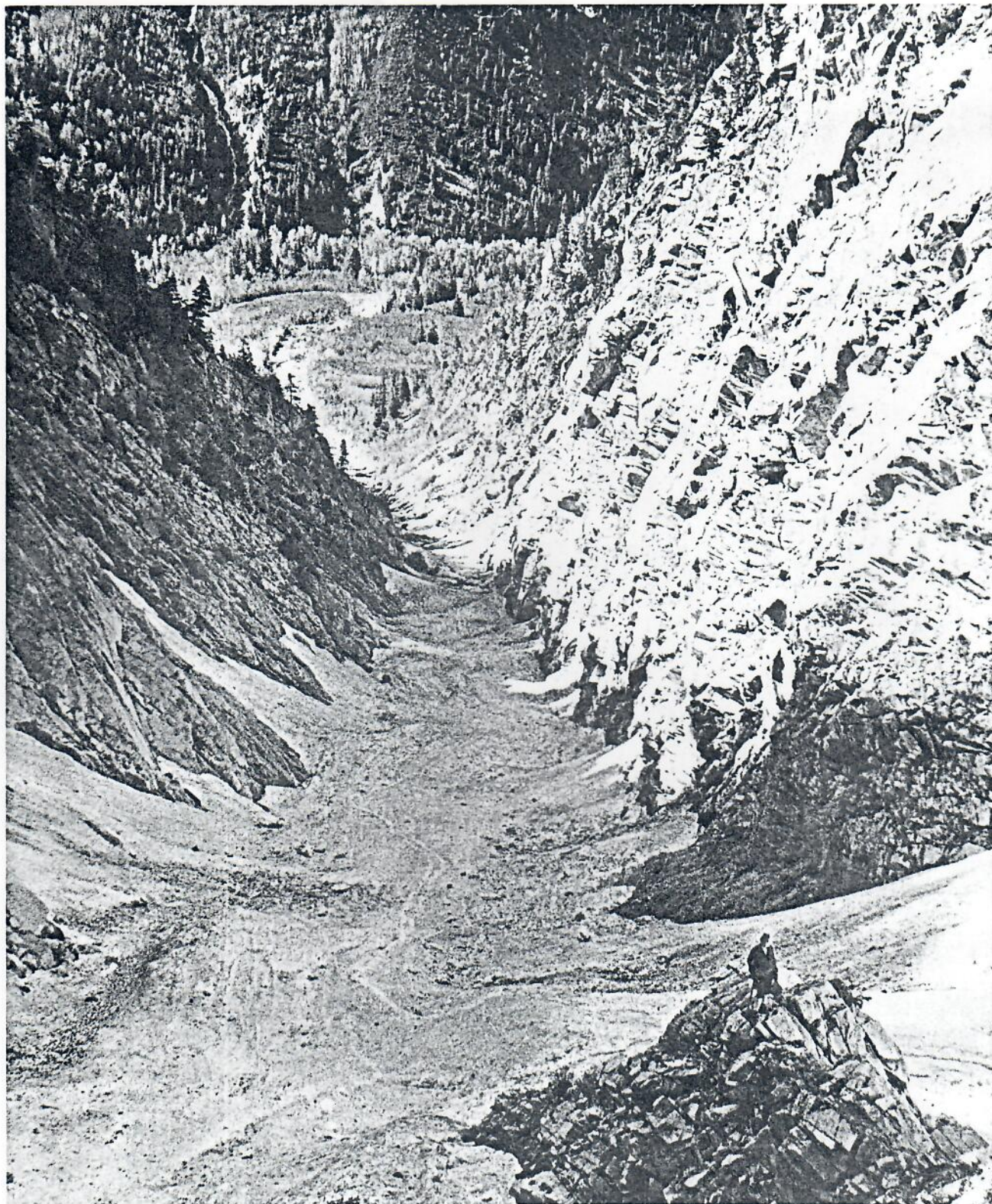
Figure 5.—View down avalanche zone of Tanner Gulch, Little Cottonwood Canyon. Barren path through young aspen growth beyond gulch defines the runout zone to where it crosses road in canyon bottom.
