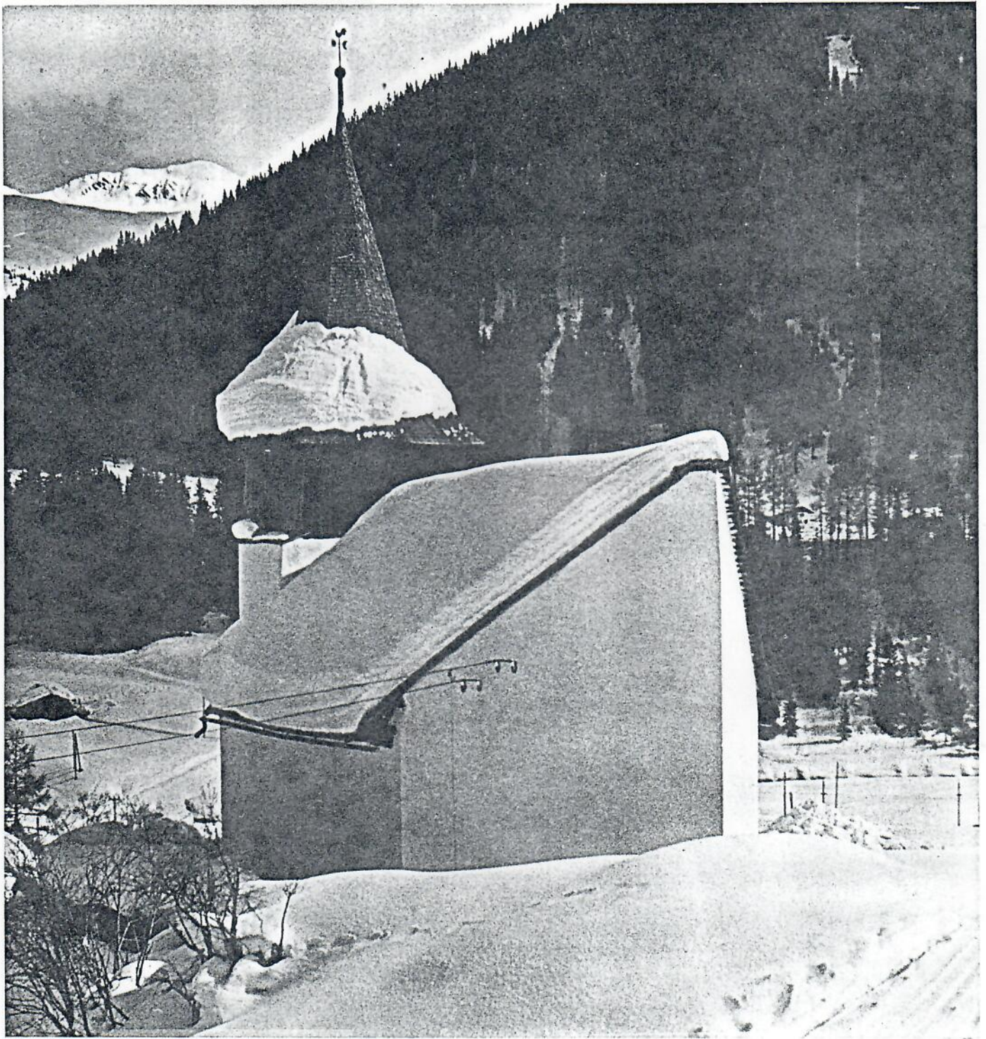
Figure 20.—Ancient Swiss church, protected by an avalanche diversion wedge. Photo, courtesy of E. R. LaChapelle.
